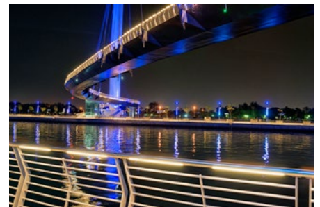
Walkway over Dubai Canal by Haralambos Parolis (25)
